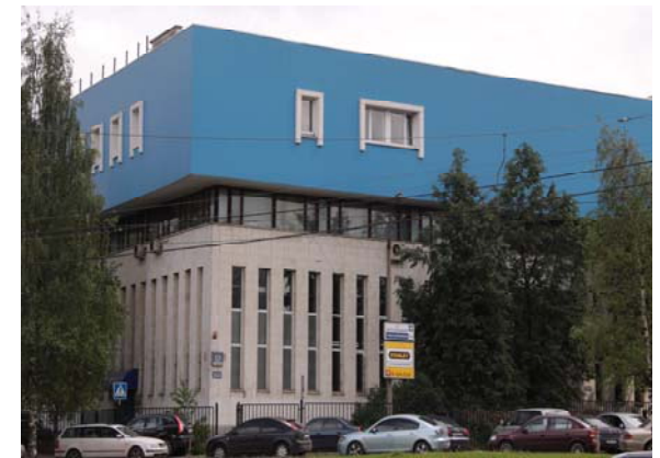
IPMech RAS building
